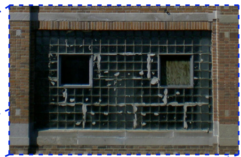
EXAMPLE OF WINDOWS TO BE REPLACED
