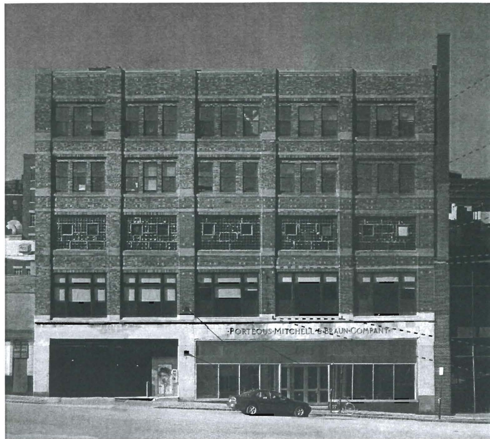
1 Photograph of Existing Free Street Elevation n/s
