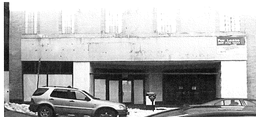
EXISTING BUILDING FRONTAGE
