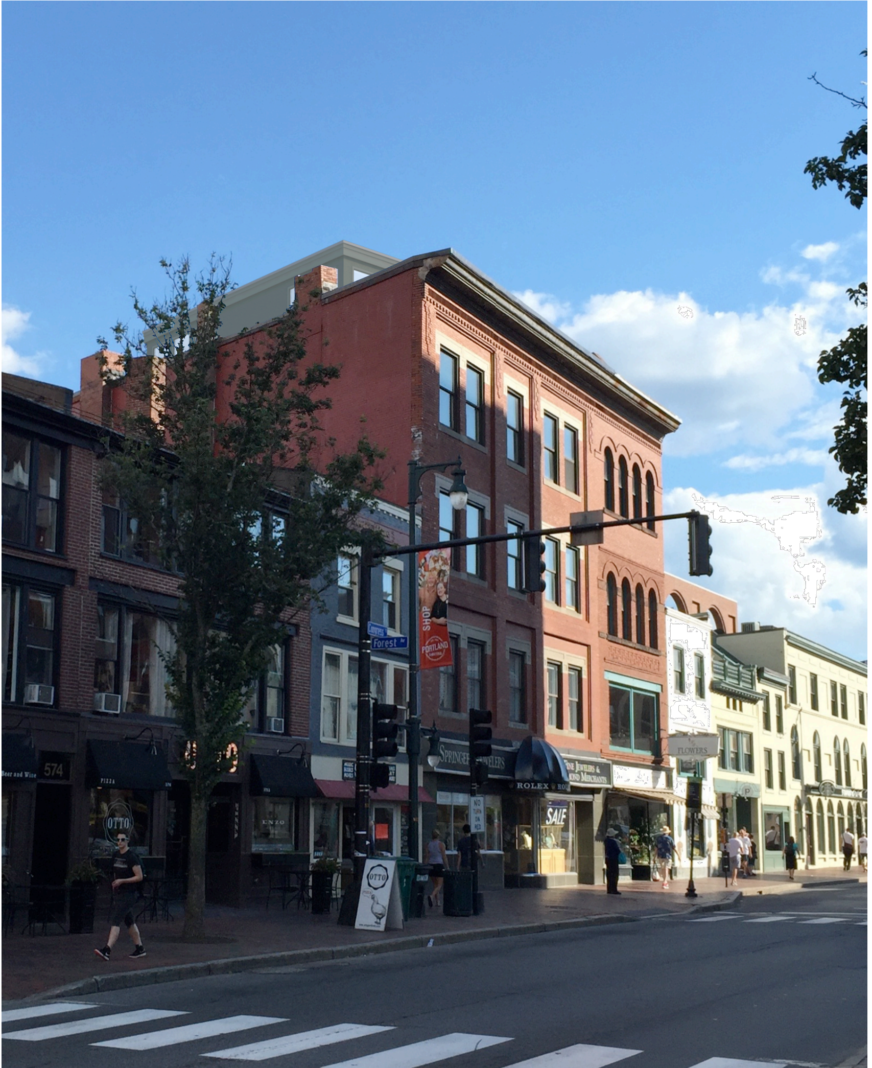
Congress Street - View from East
