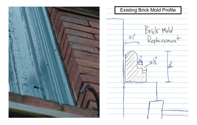
This is a basic sketch of the brick mold that we will be replacing with this project. This will be either extruded aluminum or made from wood and attached to the outside of the window frame and brick and painted.
