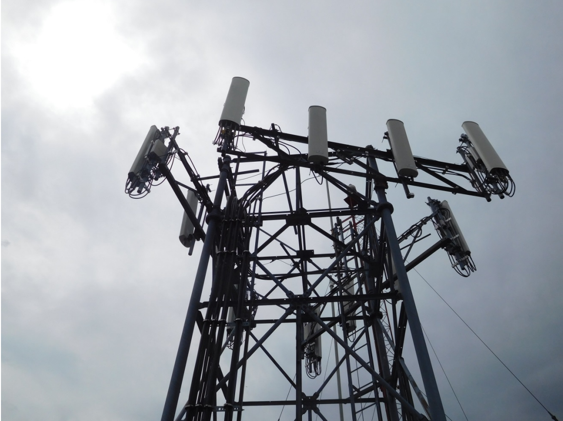
Photo 1: Photo illustrating the Tower with Appurtenances shown.
