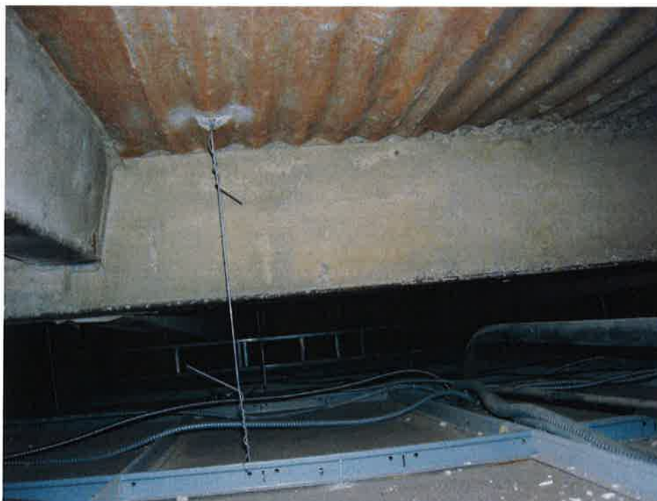
Photo 2: Sample photo illustrating the existing room floor structure.
