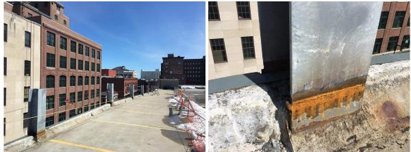
At the roof corner columns, a portion of the CMU wall removed to allow access to weld the column extensions. These blocks will need to be reinstalled prior to the installation of masonry restraint plates. (See photo below).
