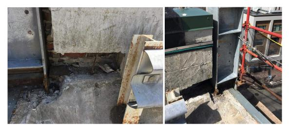
3. KISC has moved the majority of the staging from the roof to level three and completed roughly half of the brick and CMU façade demo. They anticipate completing the demo by the end of the week. (See photo below).
