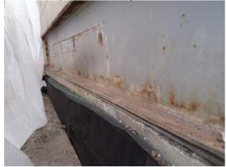
6. BSE asks that KISC rout and seal with sealant the joints between the stair CMU wall and W16 beam top and bottom flanges, see the photo above. The sealant should be compatible with the paint.
