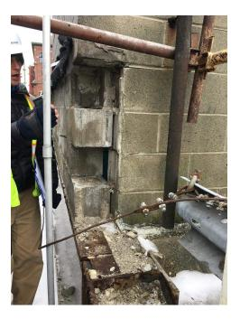
4. Where the brick masonry was removed in front of the stair tower it exposed open CMU joints and cracks that will have to be repointed. See photos below. Masonry ties should be ground flush with the CMU.
