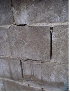
5. Step cracking in the stair tower should be repointed prior to painting of the CMU. See photo below.
