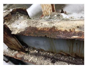
3. The existing CMU wall was toothed into the corner of the stair tower wall and KISC removed those units. See photo below. New fully grouted or solid CMU corner units will have to be reinstalled.
