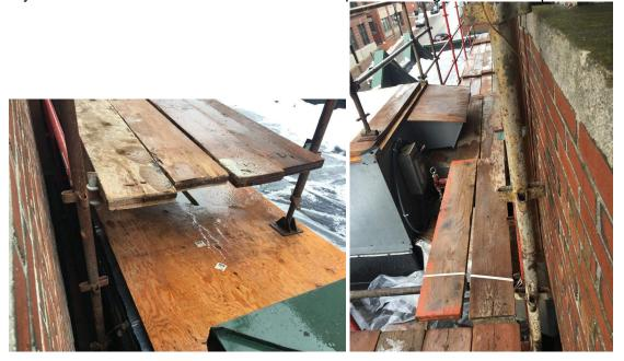
6. A staging post has been installed on the rooftop air handling unit. BSE discussed this with KISC and they noted that it will be removed. See photo above.
