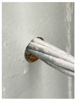
8. Each column, cable hole, and beam should be inspected for touch ups to any scratches, dings or areas missing paint. KISC is aware that final coats need to be applied to several locations at the external face of the columns. The existing "Public Parking" sign has been attached to the new steel frame, the remaining areas of the sign frame needs to be cleaned, prepped, primed and painted.
