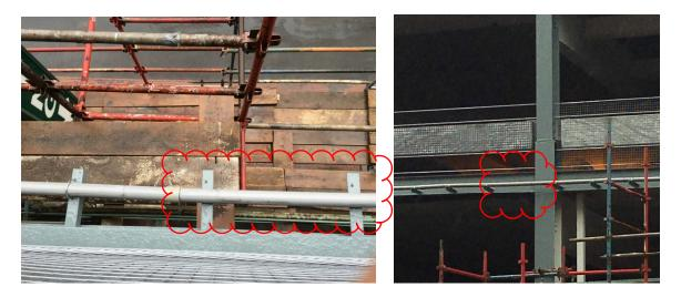
7. At the roof level, water is ponding at a pocket within the concrete curb at both sides of the column extension. KISC needs to chip away the concrete to allow the water to drain or place a sloped concrete patch, and repaint the curb. (See photo below).
