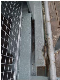
10. BSE has marked locations on the HSS bumpers with blue painter's tape where the galvanizing has been damaged. It was difficult to differentiate the difference between rust, dirt or grease so the contractor should inspect each bumper to determine if the coating needs to be repaired. (See photo below).
