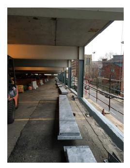
2. At level one BSE advised KISC to demolish the raised concrete curb to column line ten. The adjacent concrete curb will need to be repaired, and cold patch asphalt will be used to repair the drive surface. (See photo below).
