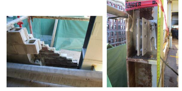
3. Due to the asphalt wash and column splice plates at level two, SCF had to raise steel clip angles for the HSS bumpers. SCF was concerned the post tension cable would be hitting the clip angle but after review of the shop drawings it appears the cable will be above the clips. (See photo above).
