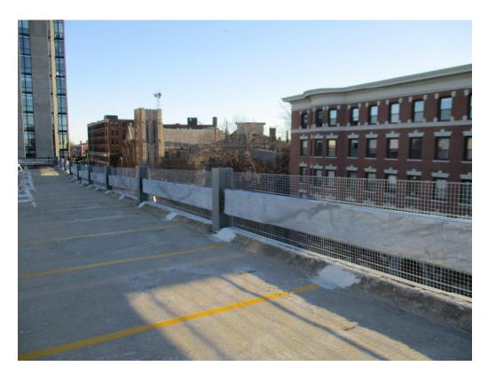
2. At level one KISC has demoed past column line 10 for access to install the HSS bumper and pedestrian cables. A portion of the CMU and brick façade will need to be rebuilt up to the column after the bumpers and cables/fencing has been installed. (See photo below).
