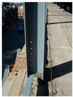
8. All HSS bumpers and clip angles for the third level façade are on site. SCF has begun installing clip angles. (See photos below).
