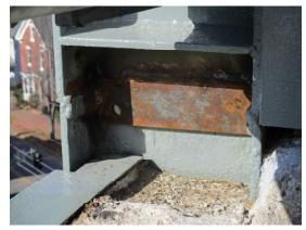
4. Rebar exposed at the concrete curb on the roof level should be ground flush with the concrete. The concrete curb is to be repaired and coated. (See photo below).
