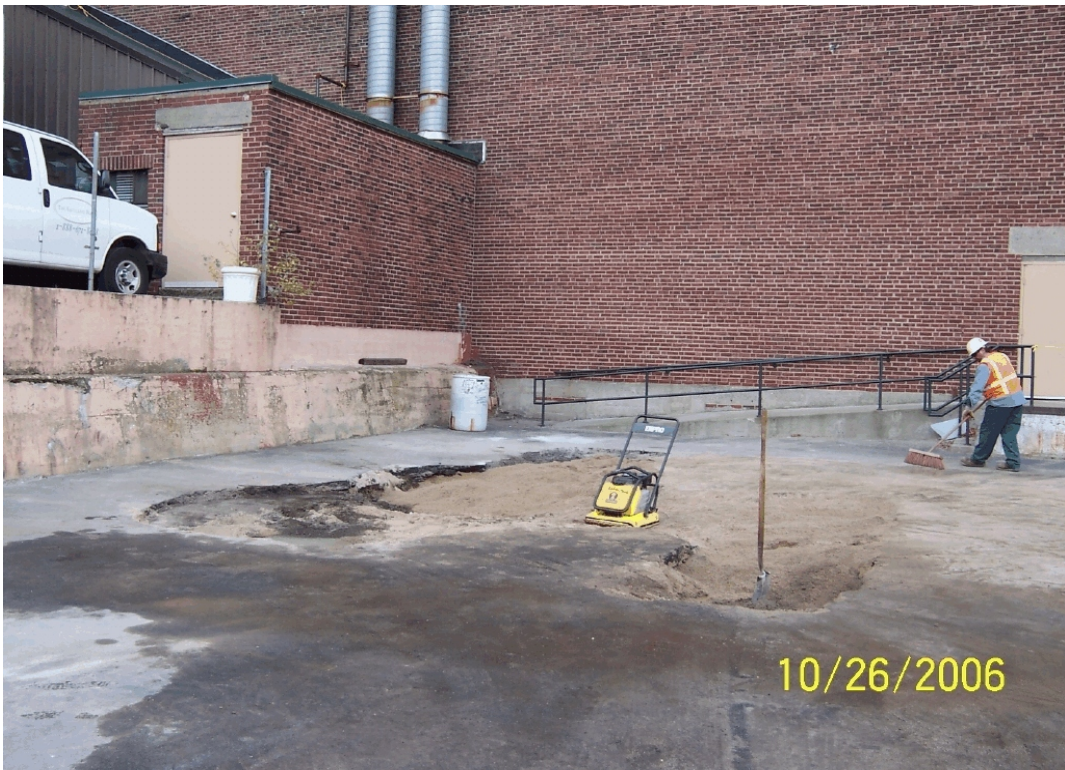
Site after filling both tanks with sand and concrete slurry.
