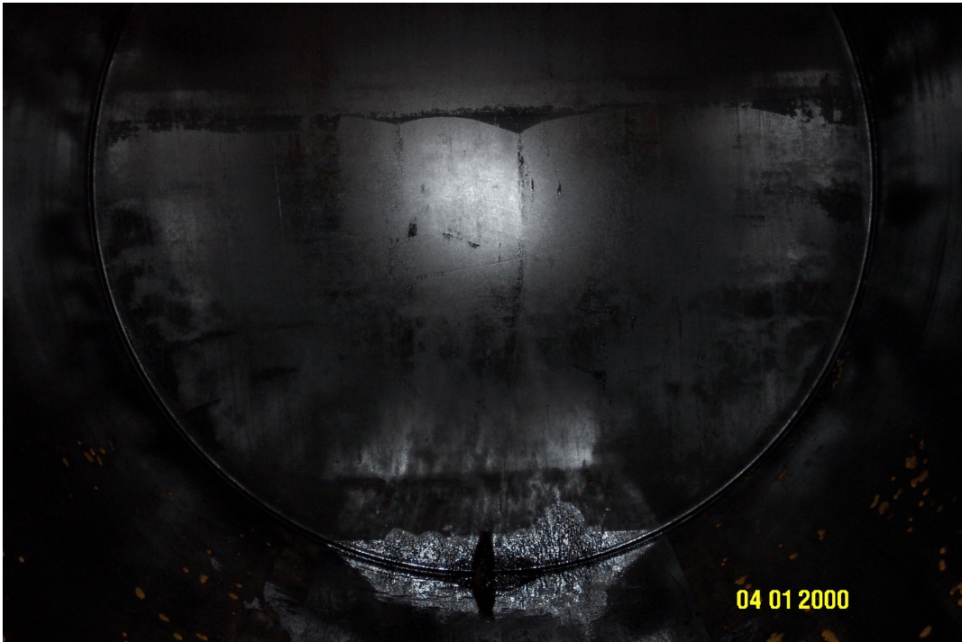
Interior of Tank #1 after cleaning. Corrosion on part of tank. (Photo date incorrect.)
