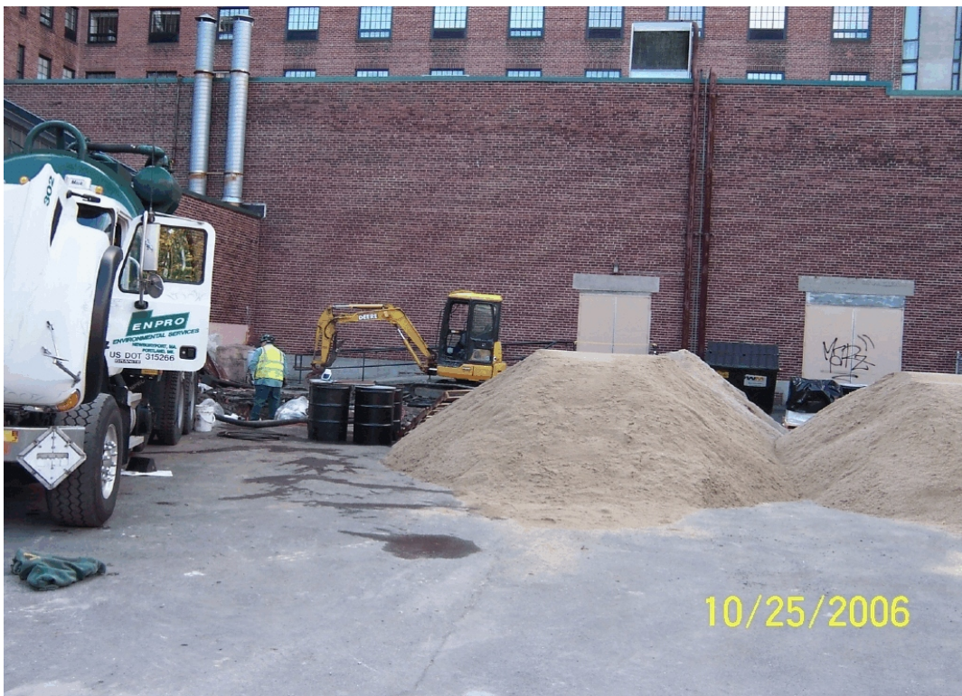
Parking Lot During Tank Vacuuming and Cleaning. Vent Pipes Already Removed.
