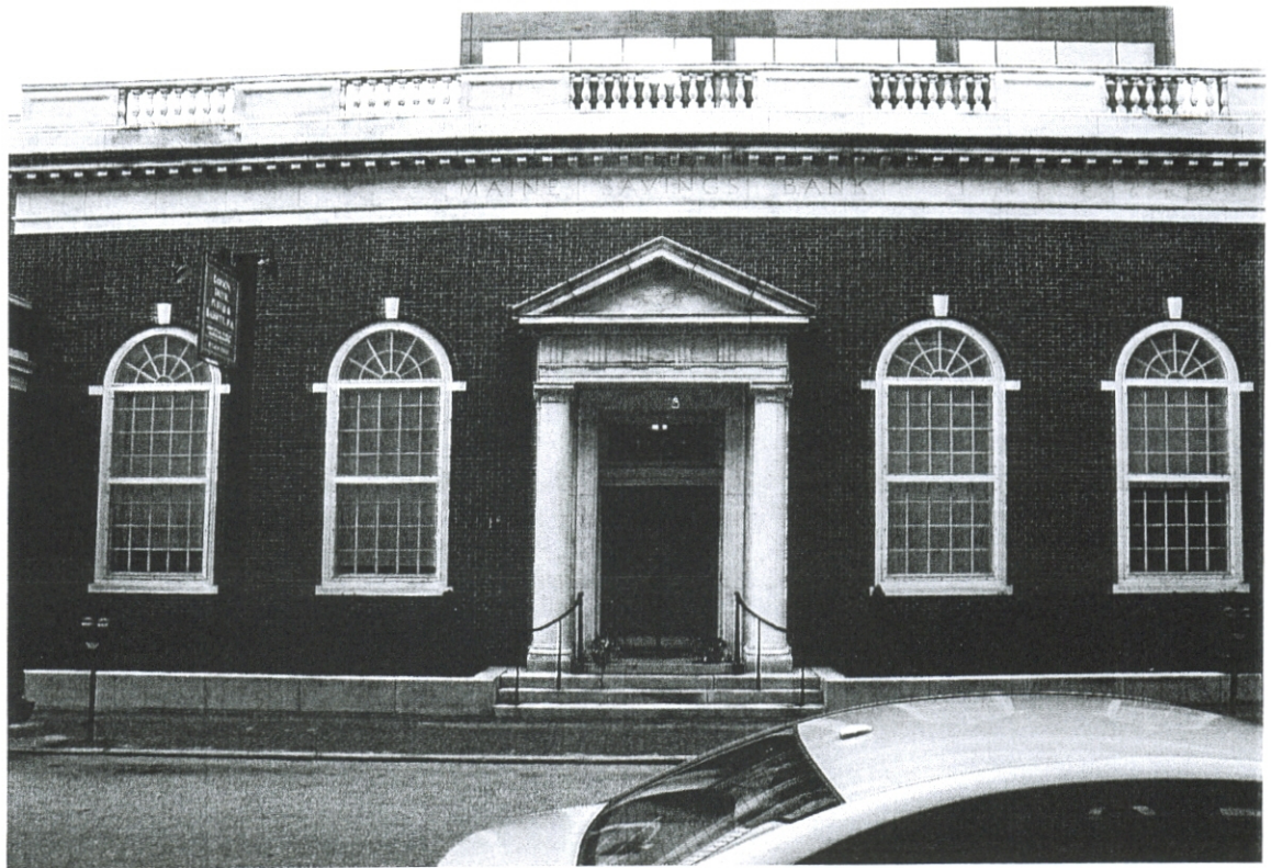
BUILDING FACADE 15 CASCO ST.
