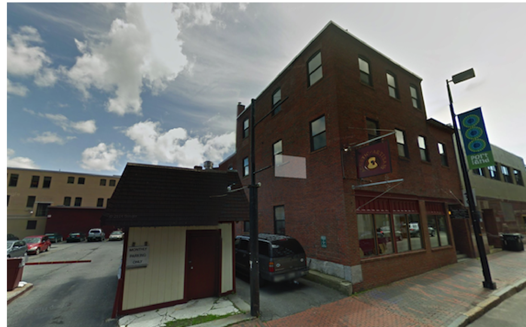
PHOTO FROM FOREST AVE LOOKING SOUTHEAST
