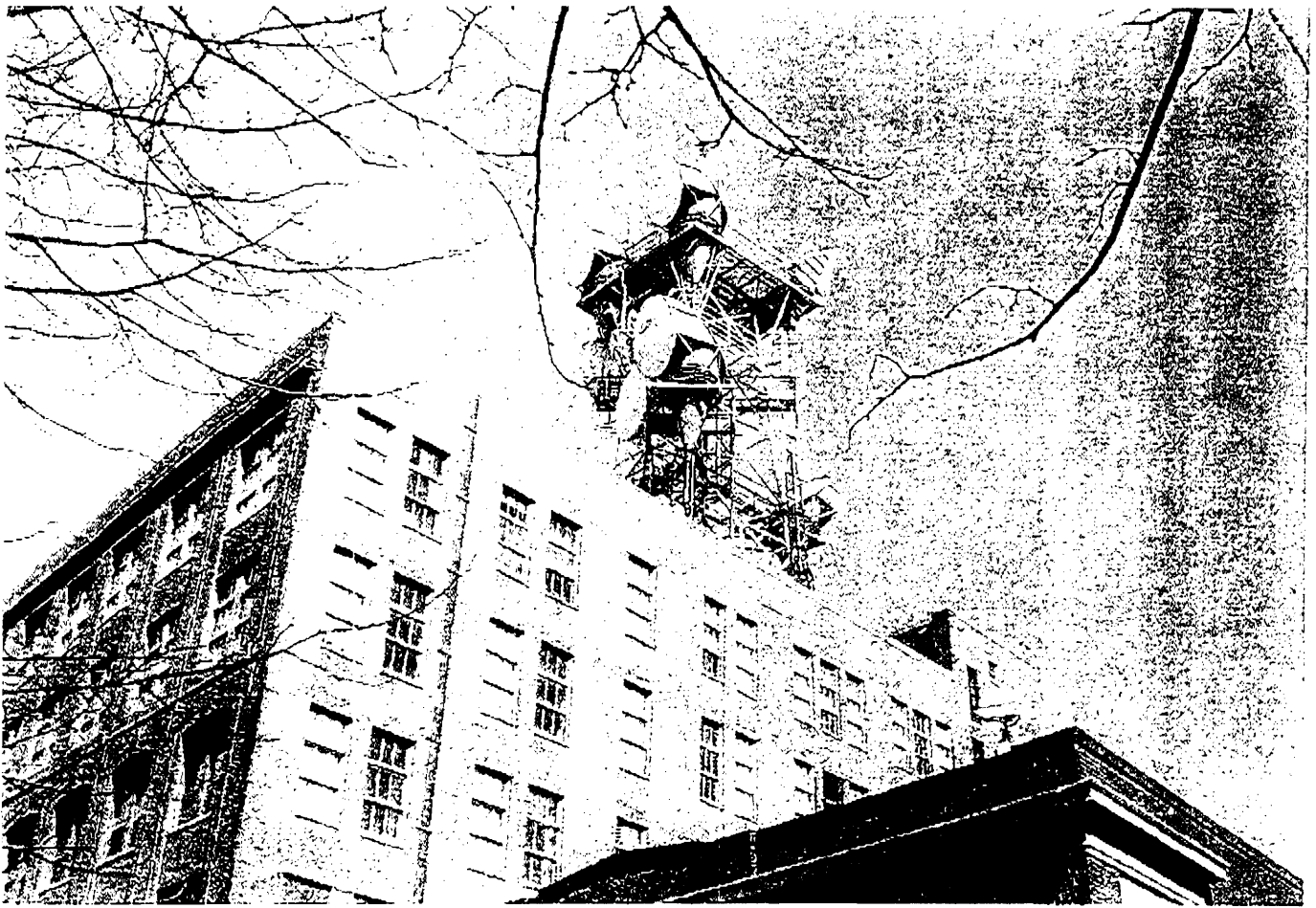
Picture 1: View of antenna and building from Forest Avenue.
