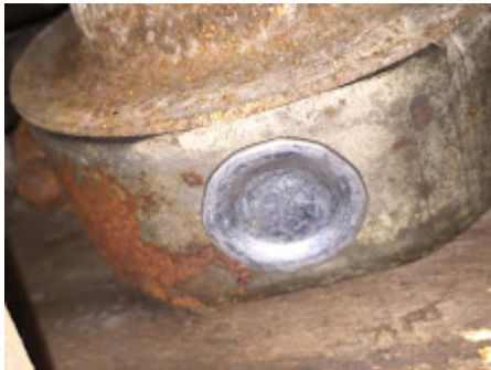
hole plug in electric box laundry room #5.jpg
