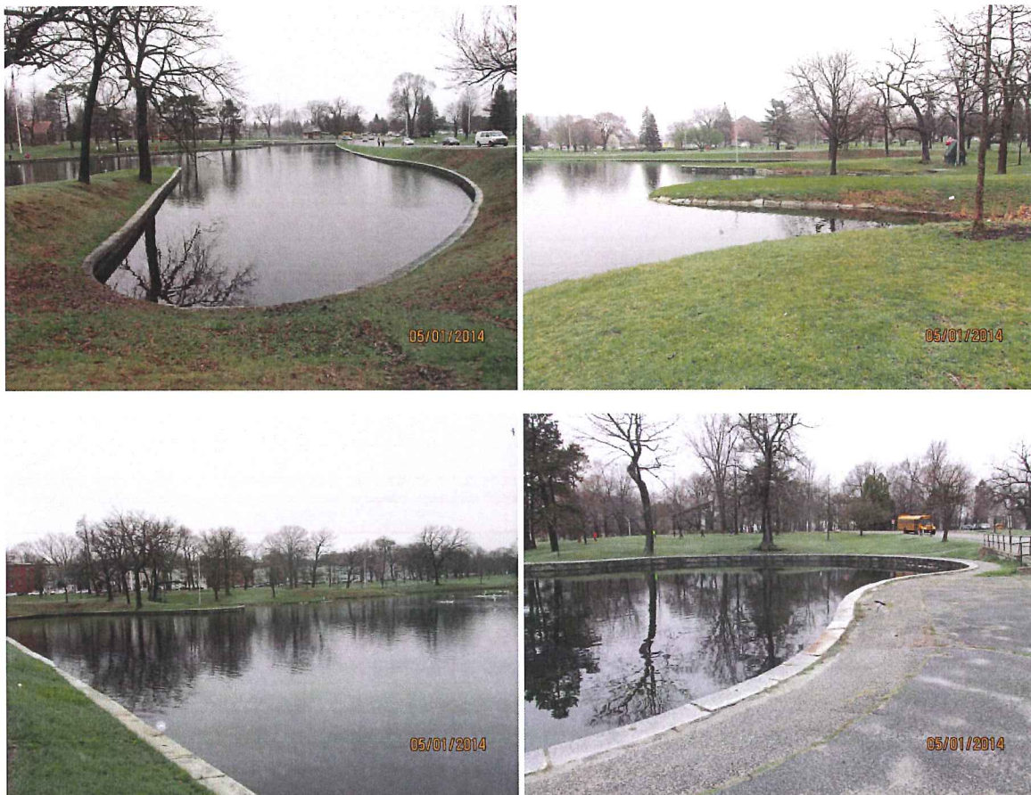
Figure 2-1 Deering Oaks Pond Existing Conditions Photographs
