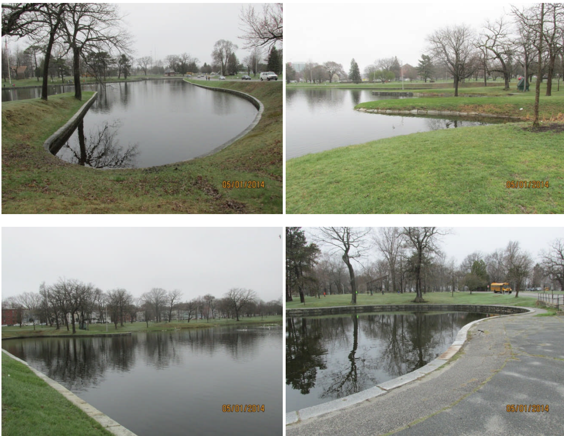
Figure 2-1 Deering Oaks Pond Existing Conditions Photographs
