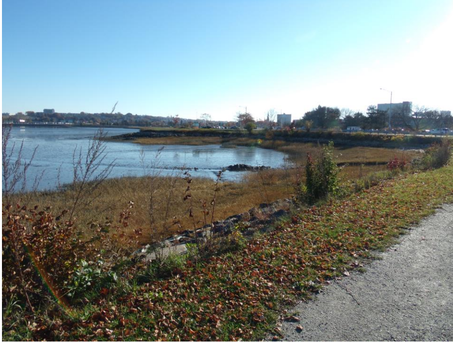
Photo 3: Looking east at the existing outfall pipe at the intersection of Baxter Boulevard, Bedford St., and Preble St. Ext.
