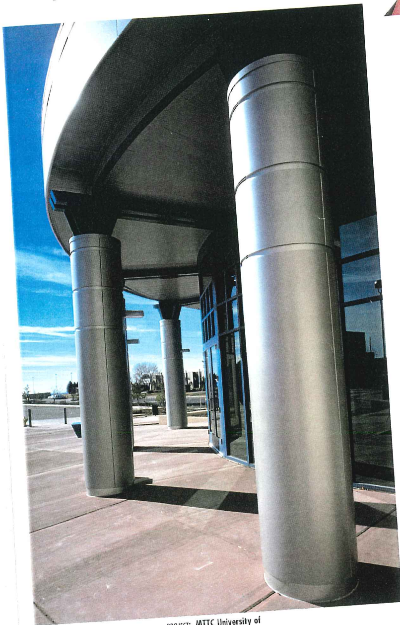
PROJECT: MITC University of New Mexico ARCHITECT: DCSW Architects, Inc. GENERAL CONTRACTOR: Gerald Martin Limited CONTRACTOR: Southwest Glass & Glazing MATERIALS: .125 Aluminum, UNA-FAB Series 200 Column Covers
