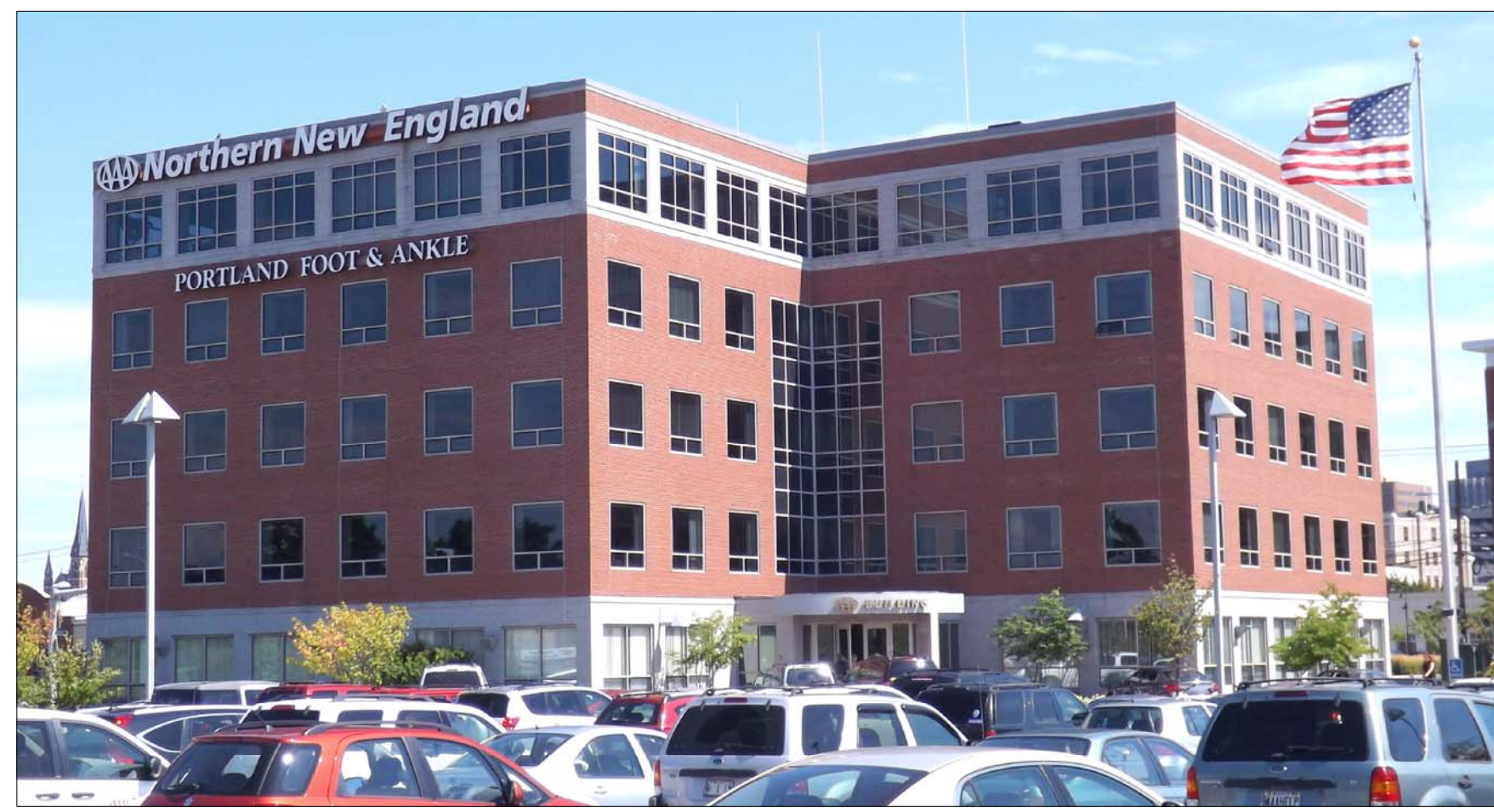
photo of building "A"
