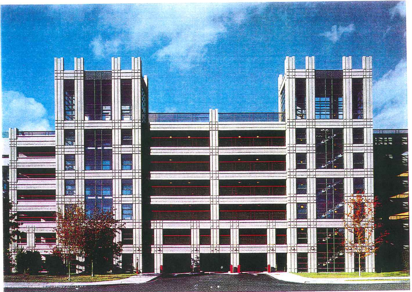
Fig. 6. Front view of parking structure shows distinctive pattern of architectural precast columns and spandrels.
