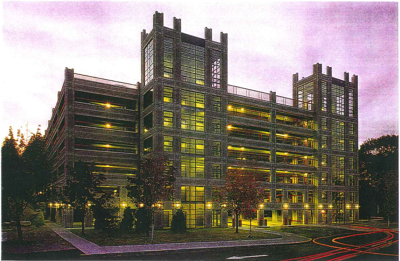
Fig. 11. Night-time view of parking structure shows how open bays, glass-encased towers, and voids create a light, airy atmosphere that reduces the building's apparent mass and gives a distinctively open feeling.
