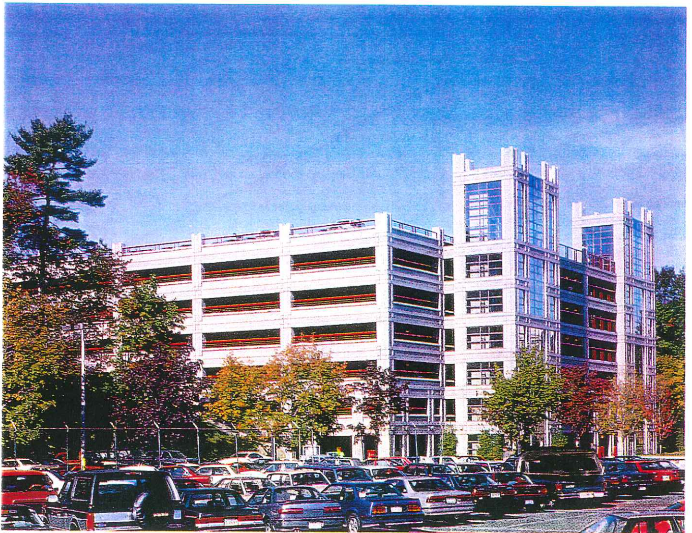
Fig. 10. Overall view of completed parking structure.
