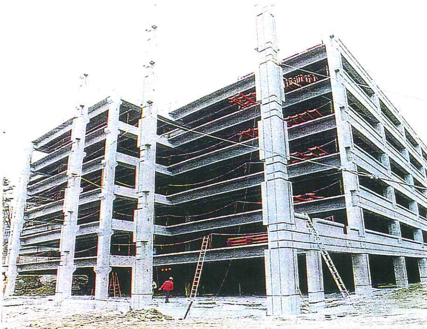
Fig. 8. Erection of precast/prestressed concrete frame of parking structure.
