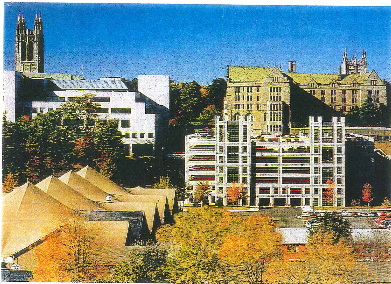
Fig. 1. The new Boston College parking structure was built into a 70 ft (21 m) hillside to create a transition space between the different styles of architecture of the lower and middle campuses.
