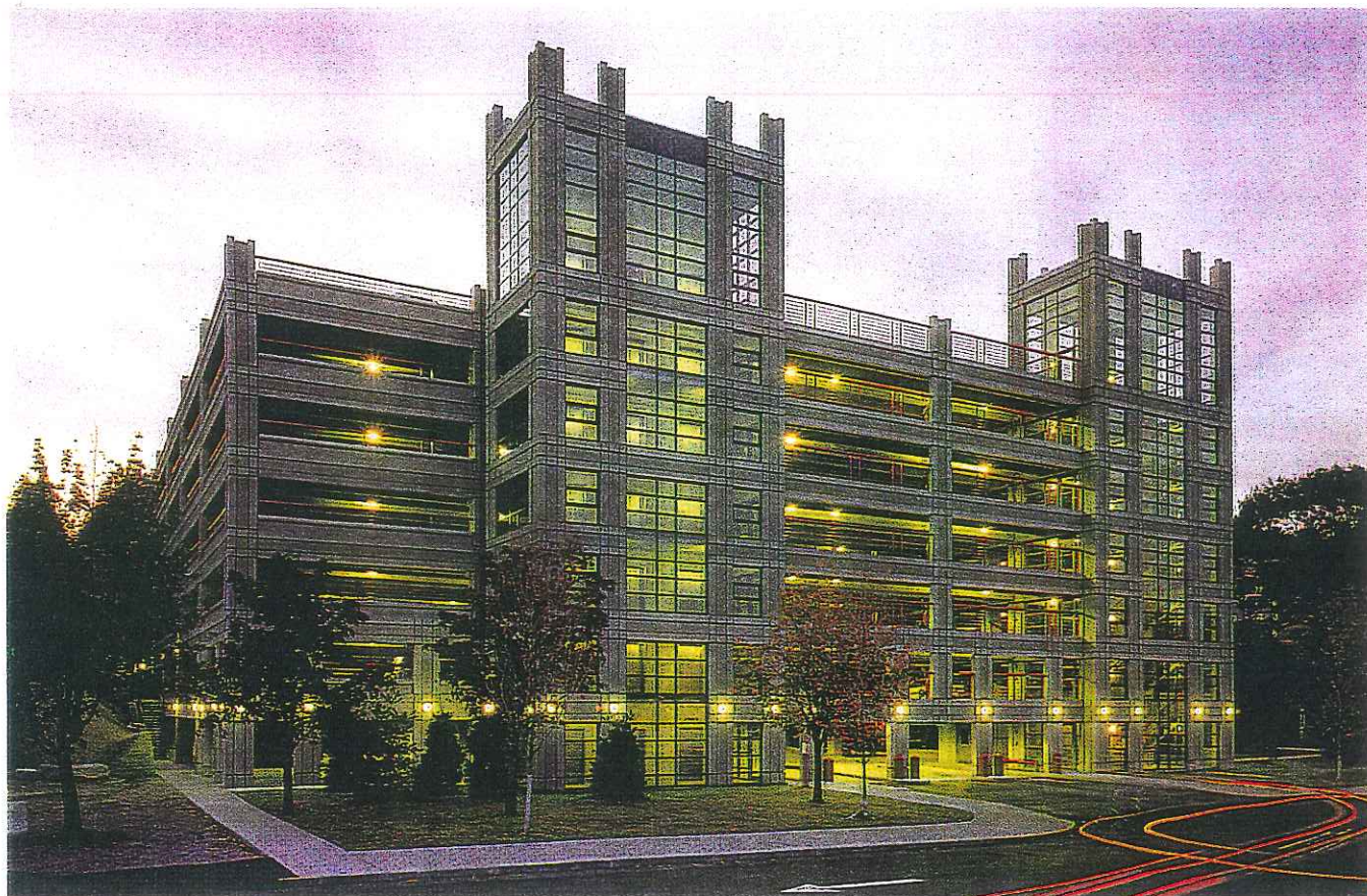
Fig. 11. Night-time view of parking structure shows how open bays, glass-encased towers, and voids create a light, airy atmosphere that reduces the building's apparent mass and gives a distinctively open feeling.
