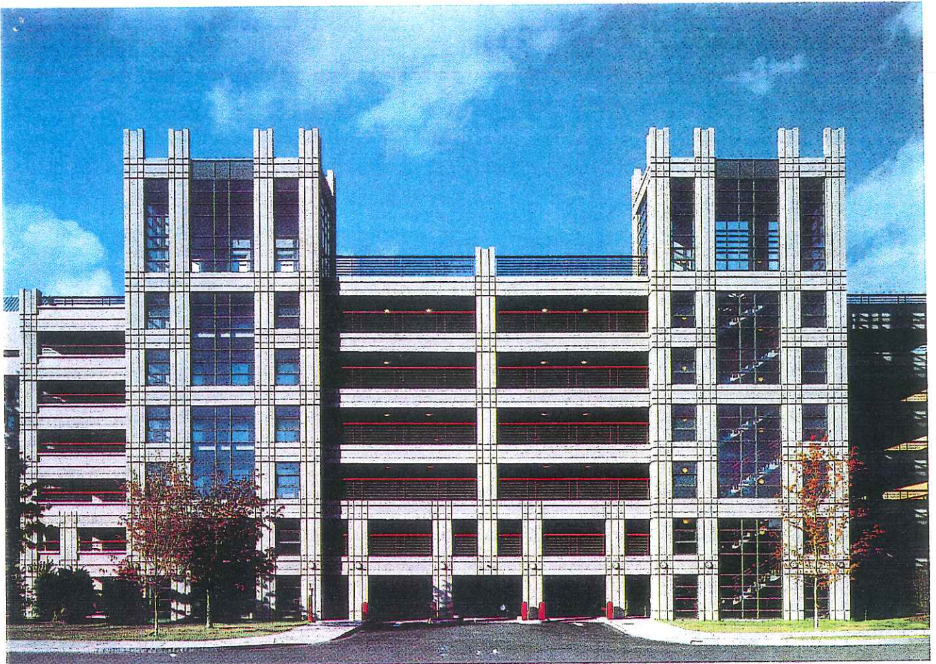
Fig. 6. Front view of parking structure shows distinctive pattern of architectural precast columns and spandrels.
