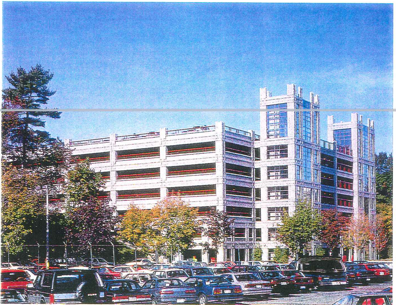
Fig. 10. Overall view of completed parking structure.
