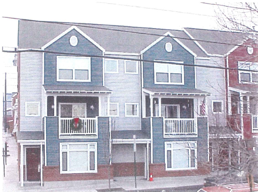
Unity Village on Stone Street and Cumberland Avenue
