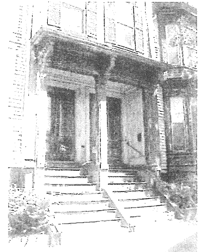
House in need of repair
