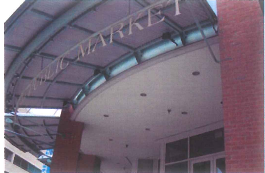
EXISTING CANOPY DOWN-LIGHTS
