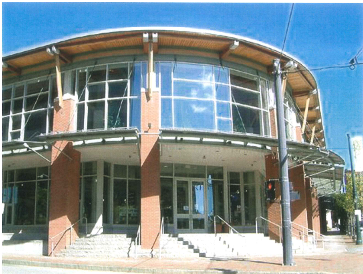
EXISTING ENTRANCE AT THE CORNER OF CUMBERLAND AVE. AND PREBLE ST.
