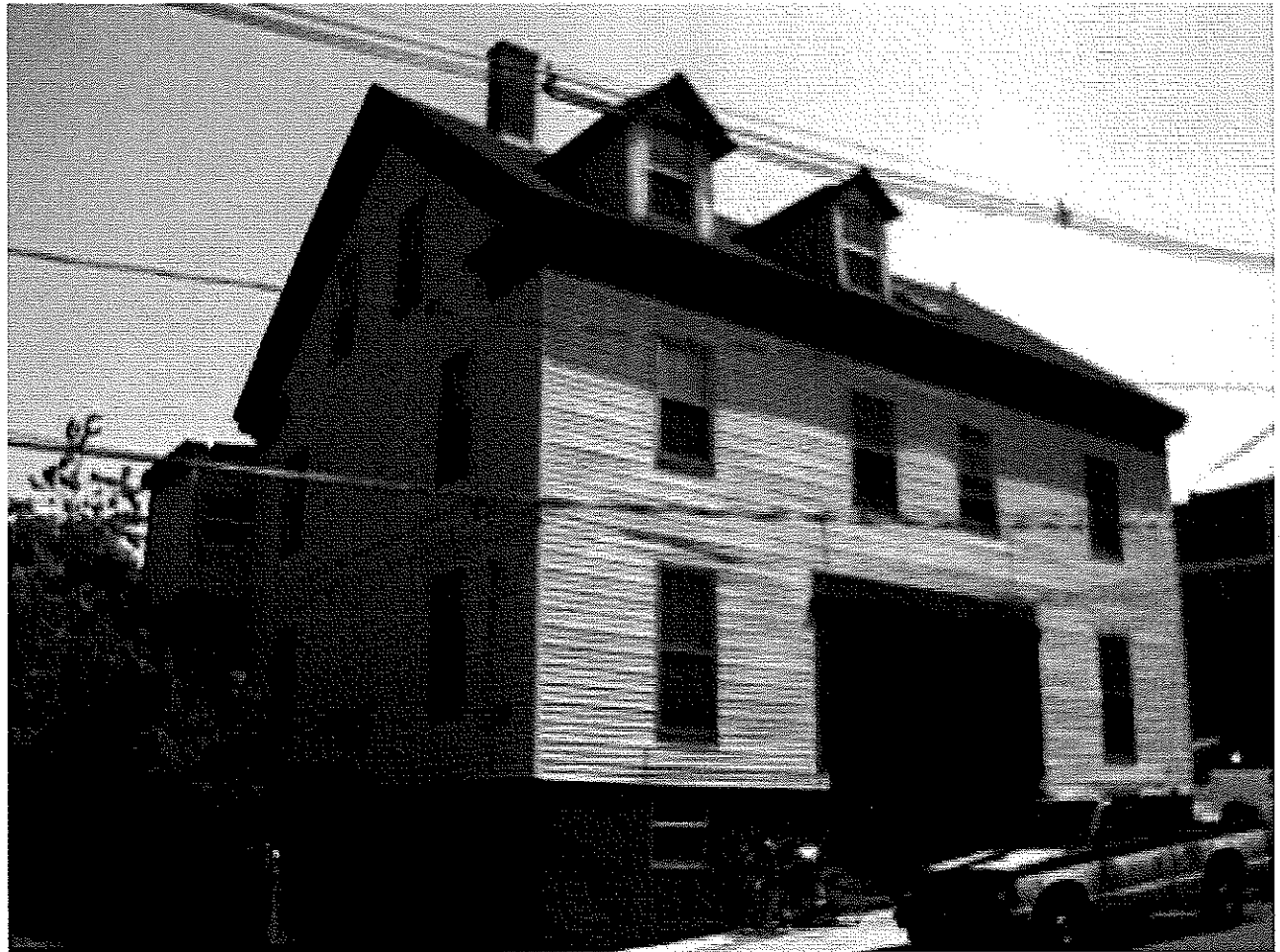
Front of Building
