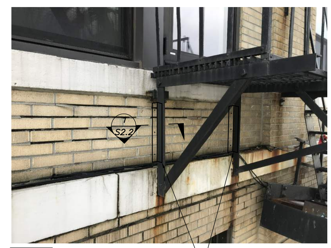
PHOTO 1 NEW STEEL ANGLES WITH ANCHORS TO BRICK MASONRY (SEE SECTION)
