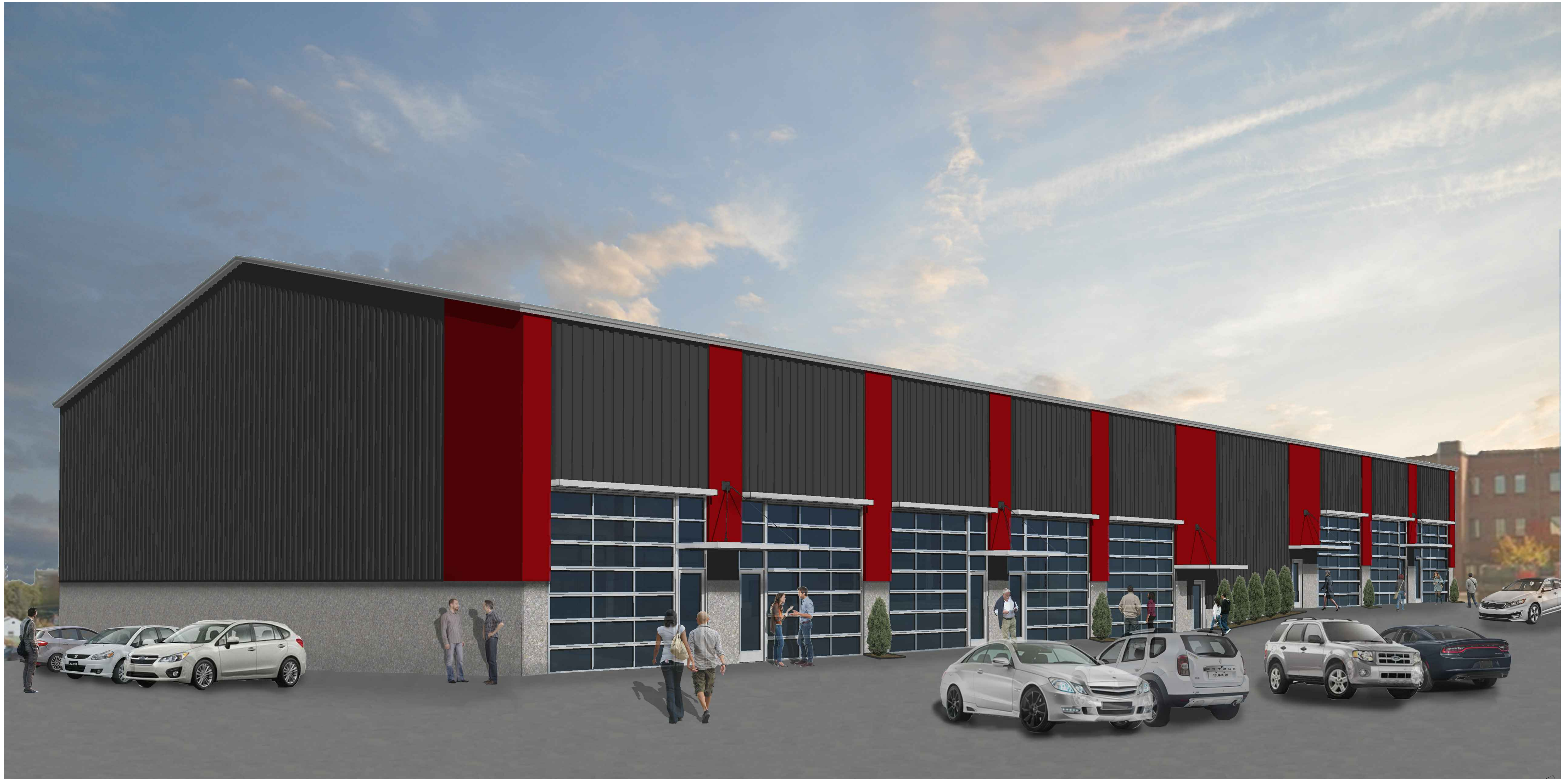
1 VIEW LOOKING SOUTH-EAST ON PARRIS STREET N.T.S.
