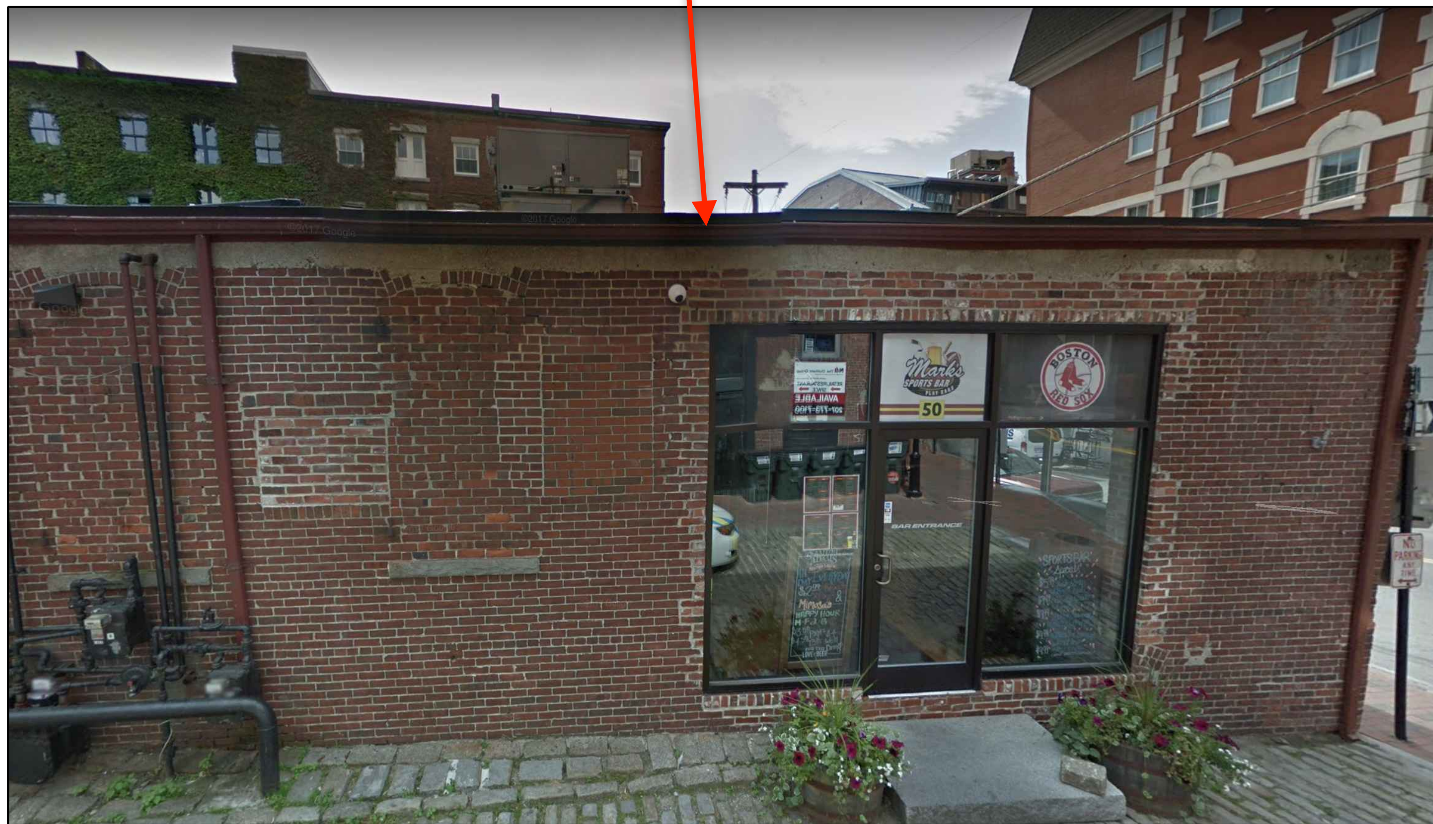
3 EXISTING VIEW LOOKING SOUTH ON WHARF STREET
