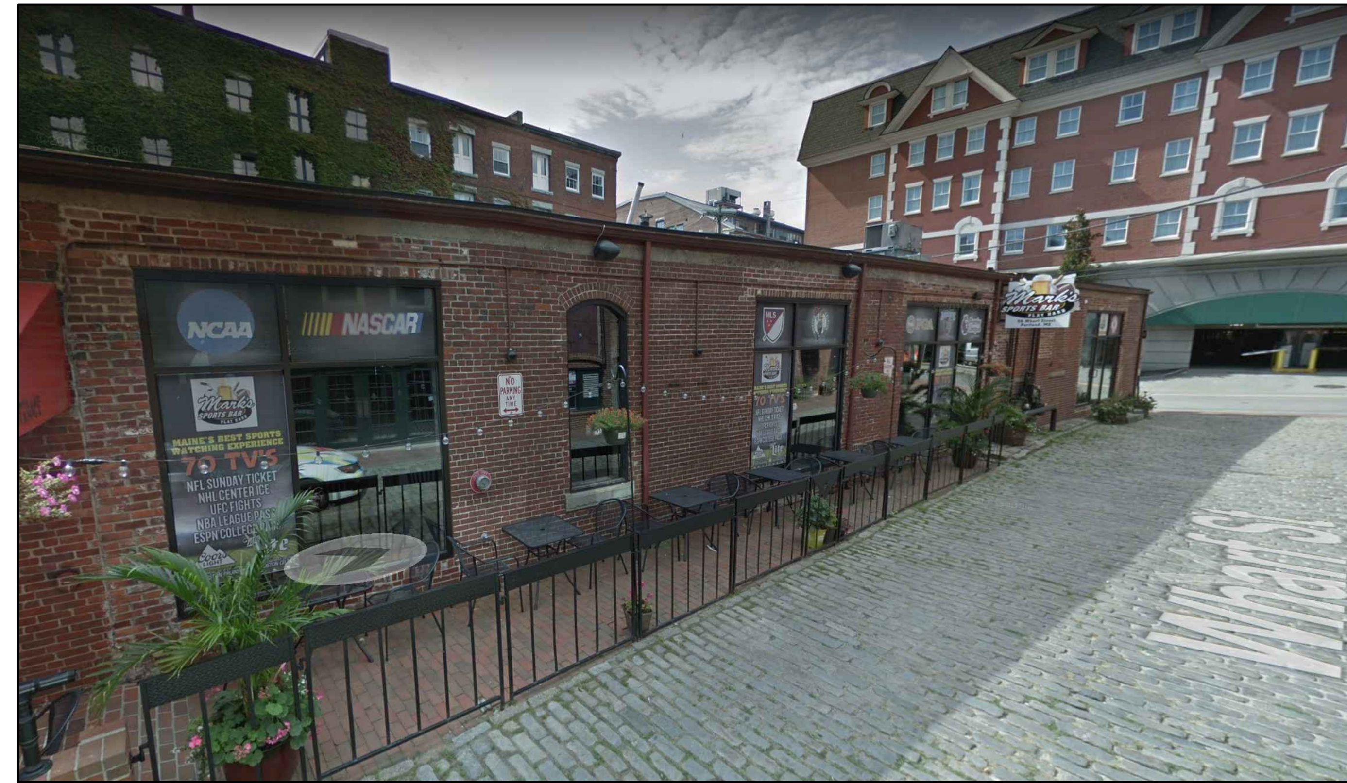
2 EXISTING VIEW LOOKING WEST ON WHARF STREET
