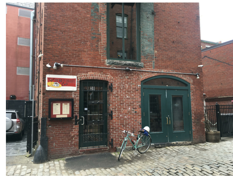
EXISTING FACADE PHOTOGRAPH (MAY 2017)
