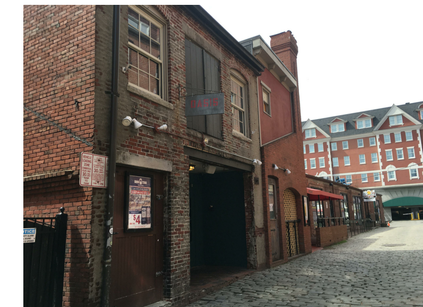
SITE CONTEXT | BUILDINGS W/ADJACENT BLOCK ALONG WHARF STREET
