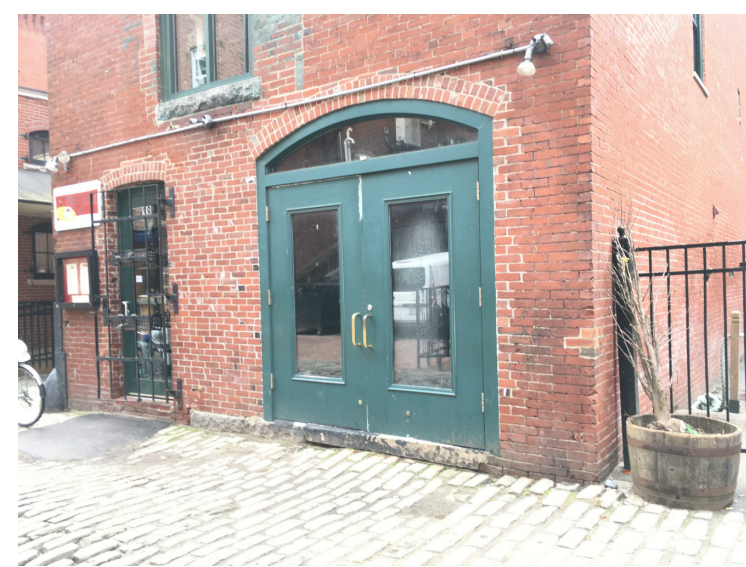
EXISTING FACADE PHOTOGRAPH (MAY 2017)
