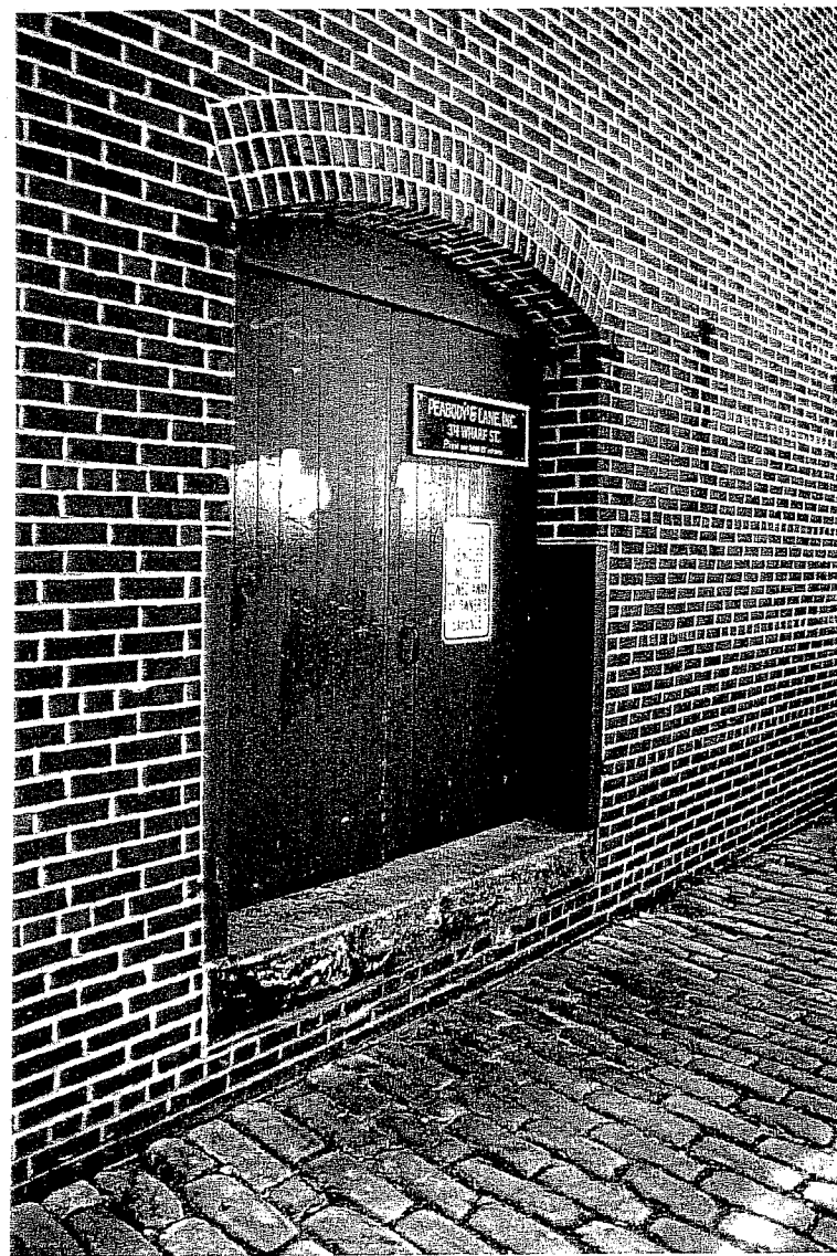
OPENING ON WHARF ST TO BE GLAZED IN
