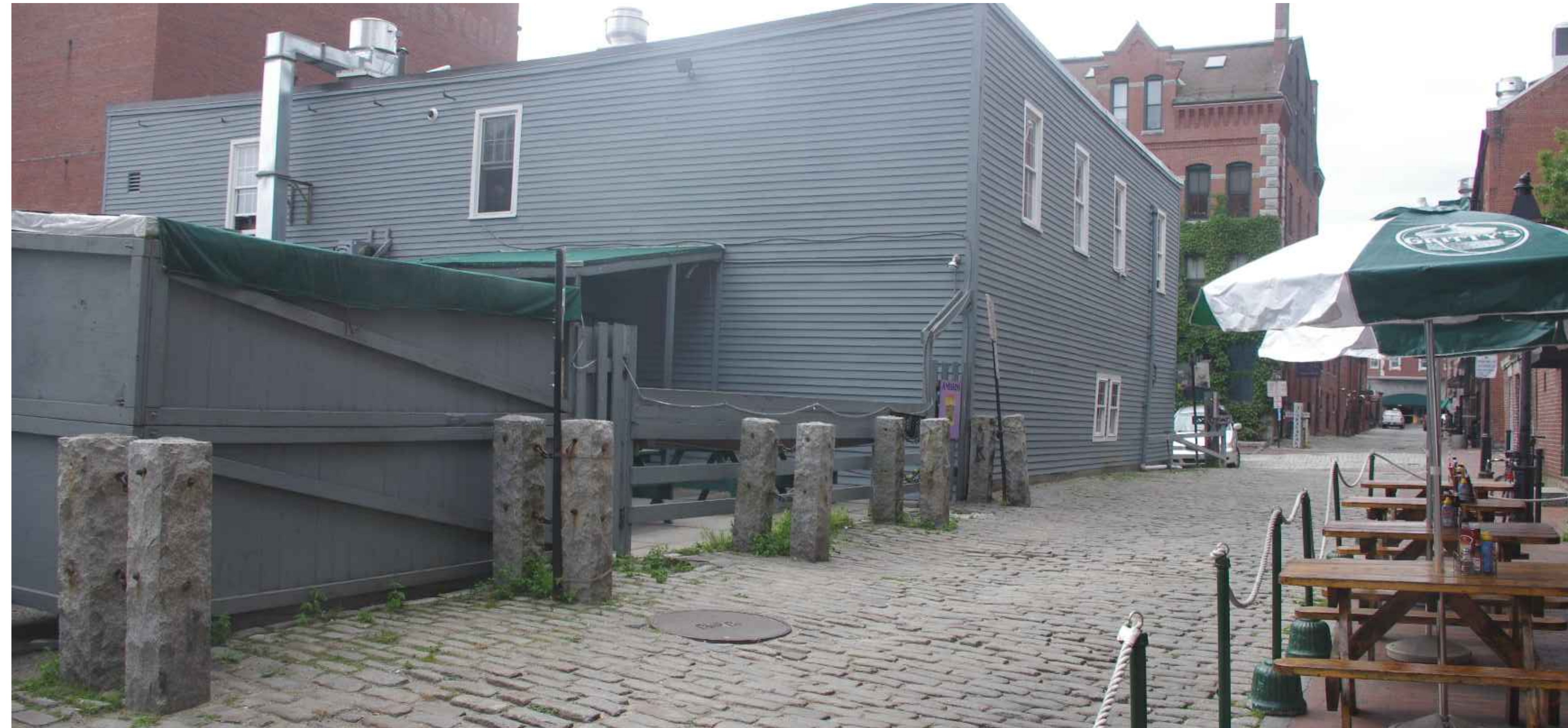
1a Existing view from Wharf Street, looking South NTS
