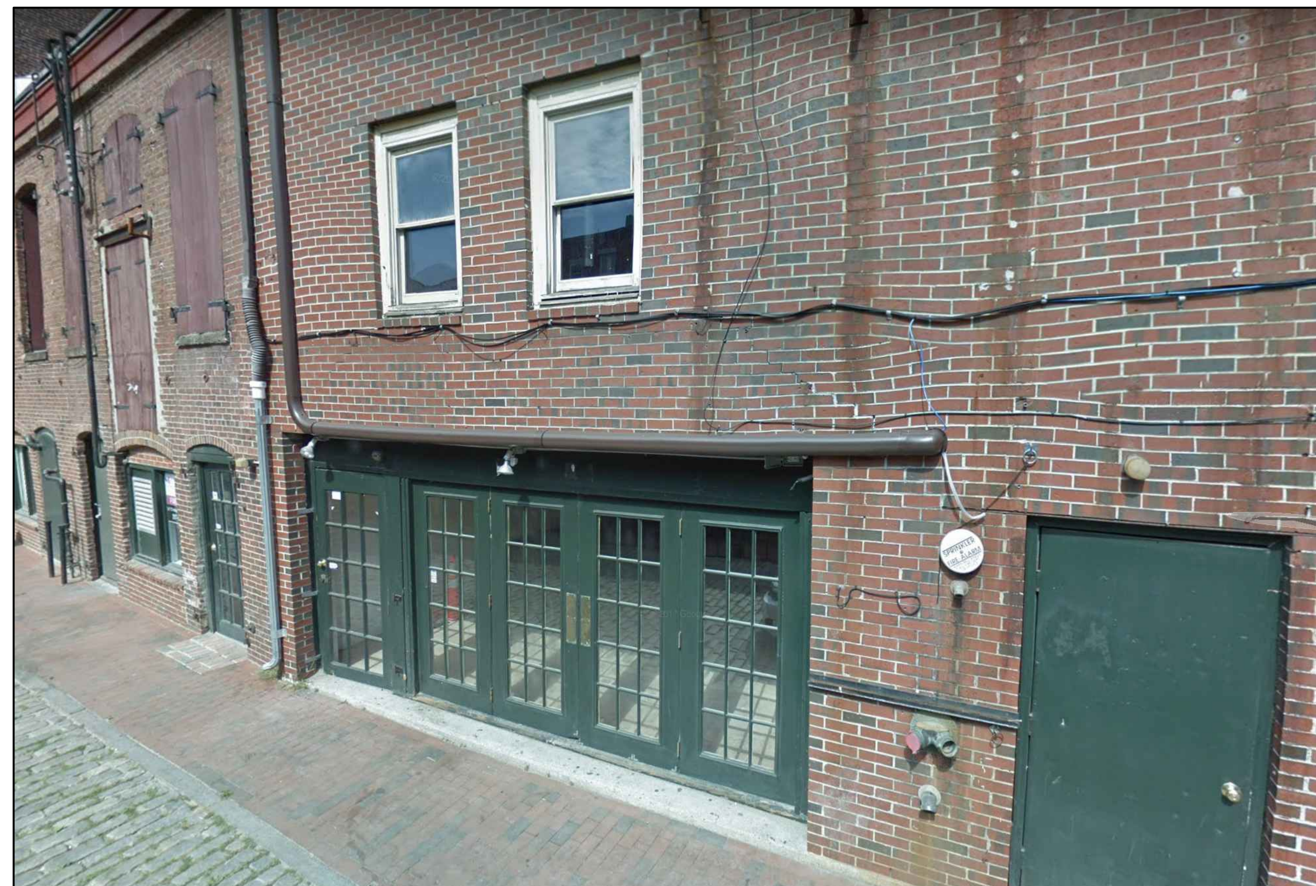
1 VIEW OF 51 WHARFEXISTING MULTI-LEAFDOORS
