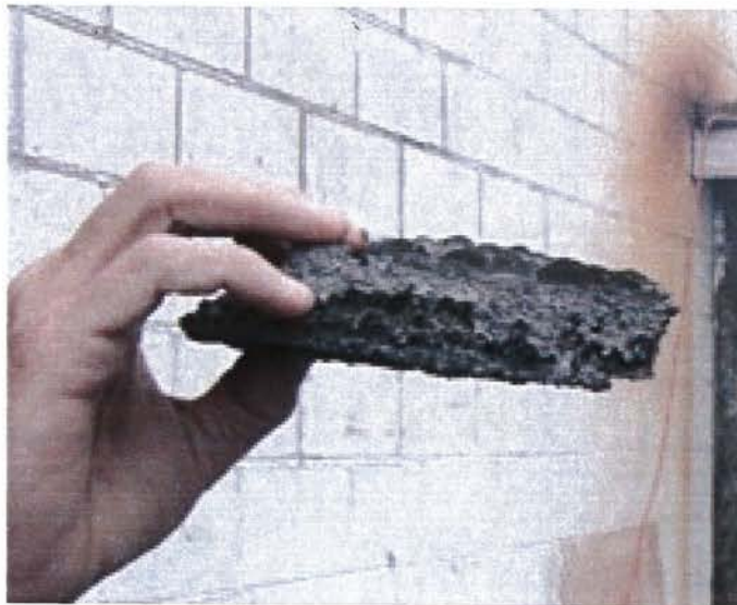
Illustrating thickness of intumesced coating
