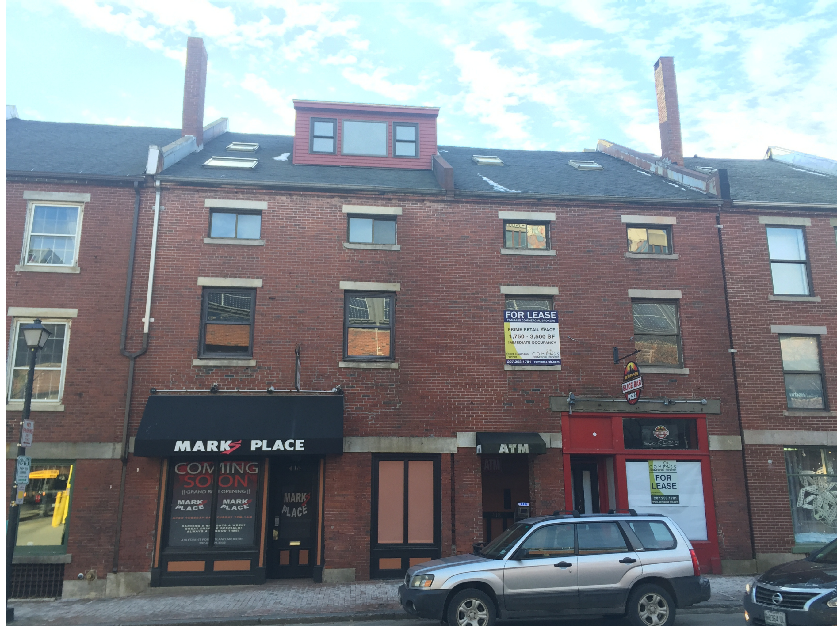
FORE STREET EXISTING
