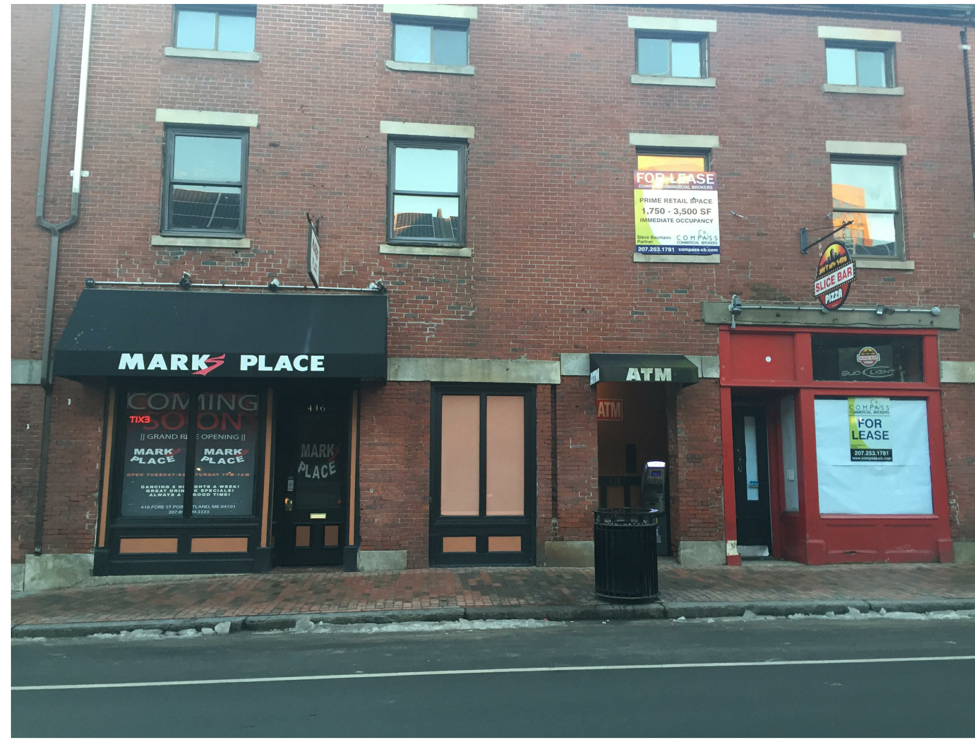
FORE STREET - EXISTING
