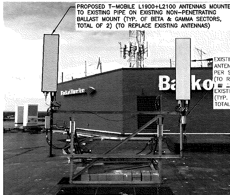
T-MOBILE ELEVATION PHOTO DETAIL (BETA & GAMMA SECTORS)
