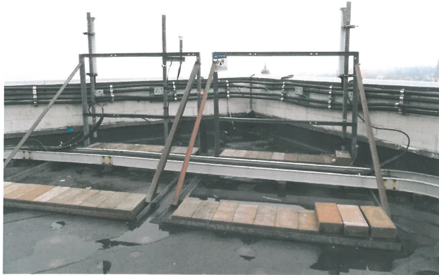
Photo 1: Sample photo showing the existing antennas.
