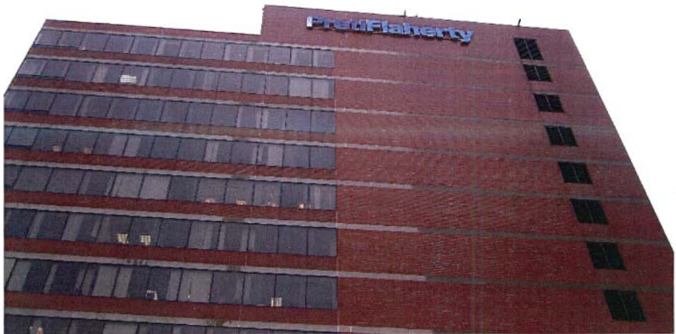
Top of Temple Street Facade
