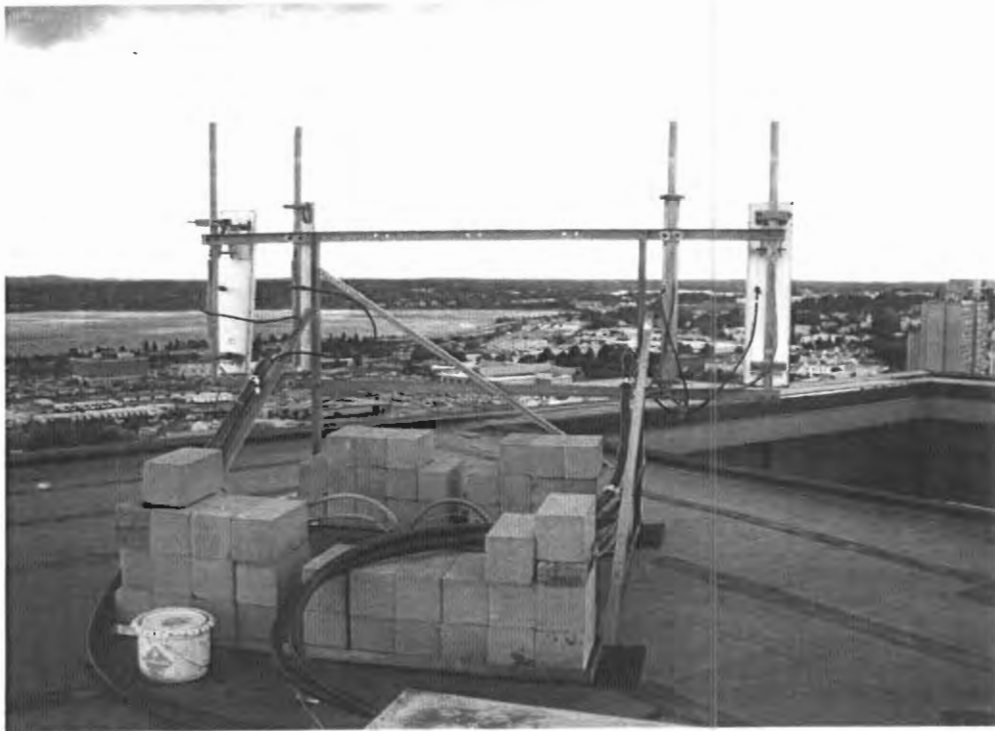
Photo 1: Sample photo of the existing Verizon Antennas secured to the existing roof top sled mount.
