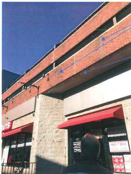
Image-05 Fore Street facade showing the deterioration of brick and stalactites formed from years of moisture and salts seeping from masonry.
