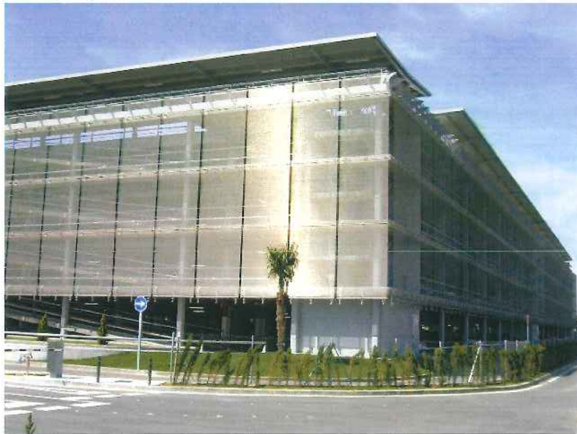
Image-07 Demonstrates the material's translucent properties that screen but do not conceal the parking garage.
