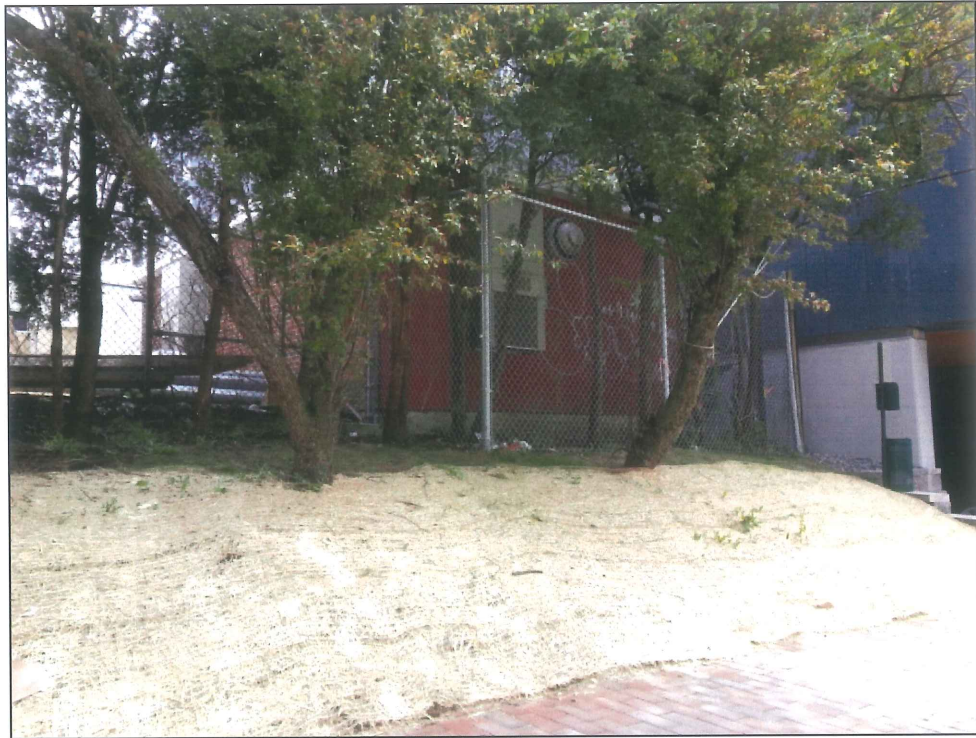
Photo 1. Chain link fence to be replaced with erosion controls in place between the existing landscaping and the sidewalk.
