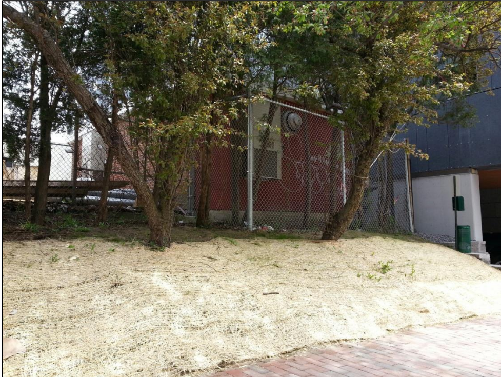
Photo 1. Chain link fence to be replaced with erosion controls in place between the existing landscaping and the sidewalk.
