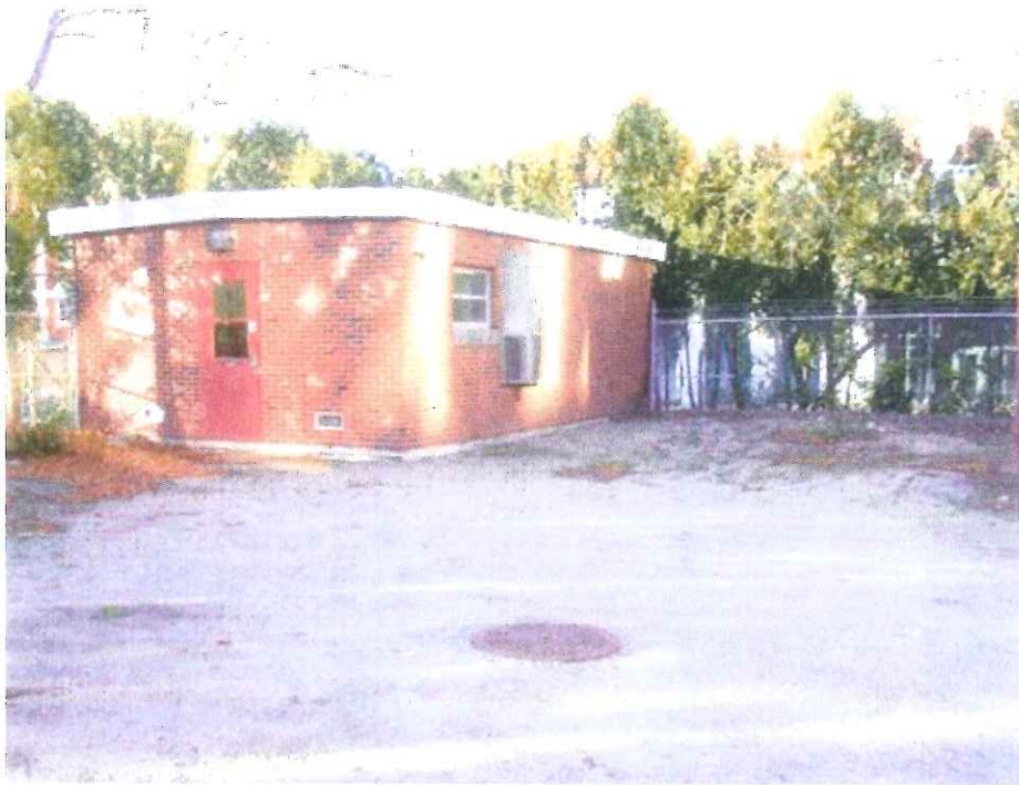
Photo 1. Control house to remain.
