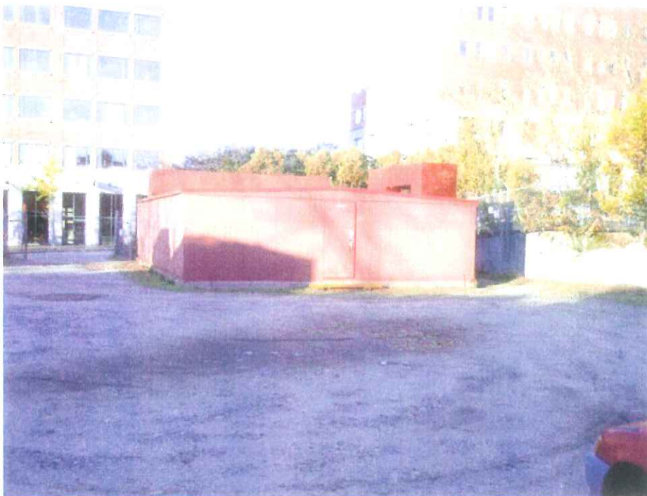
Photo 2. Existing 34.5 kV switchgear to be replaced with a similar 11.5/12 kV switchgear.
