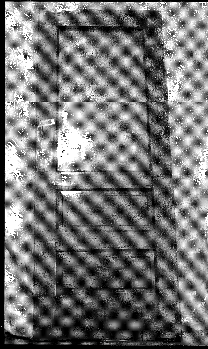
FR DOOR # 19 DOOR THICKNESS 1-3/8" DOOR WIDTH 30-1/8" DOOR HEIGHT 81-1/2"
