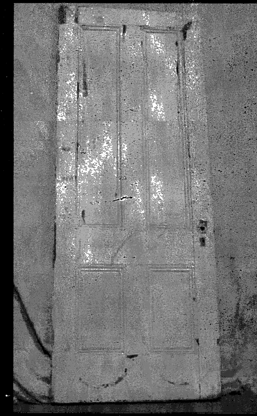
FR DOOR # 17 DOOR THICKNESS 1-3/4" DOOR WIDTH 31-5/8" DOOR HEIGHT 83-3/8"
