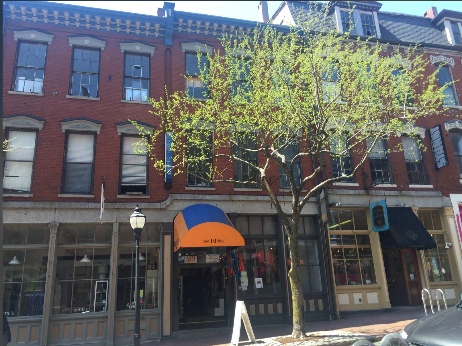
10 Exchange Street – Exchange Street Existing Facade
